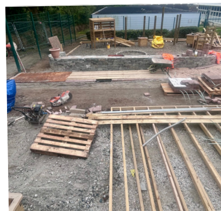
Ground and preparation work on the outside space
